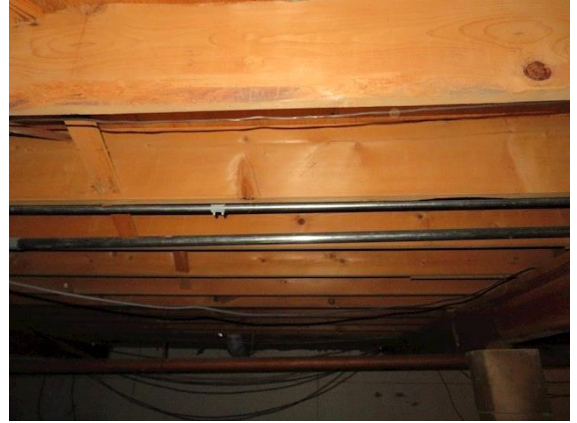
Under Floor Framing & Support:
