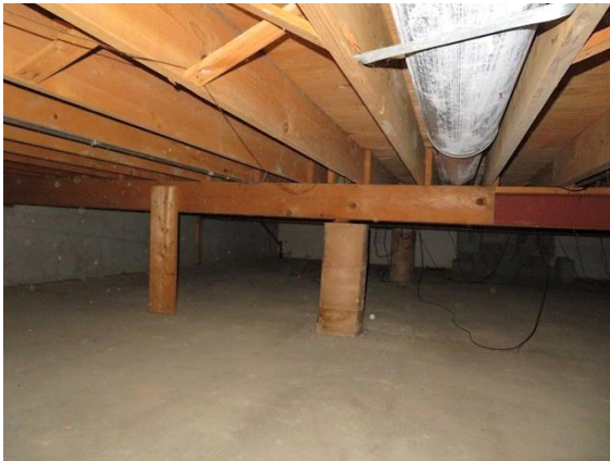
Under Floor Framing & Support:
