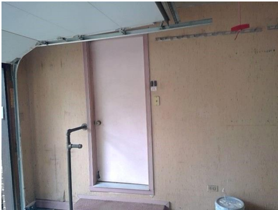
Garage Pedestrian Door into House:
