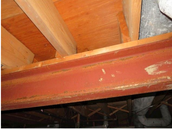
Under Floor Framing & Support:
