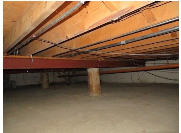
Under Floor Framing & Support:
